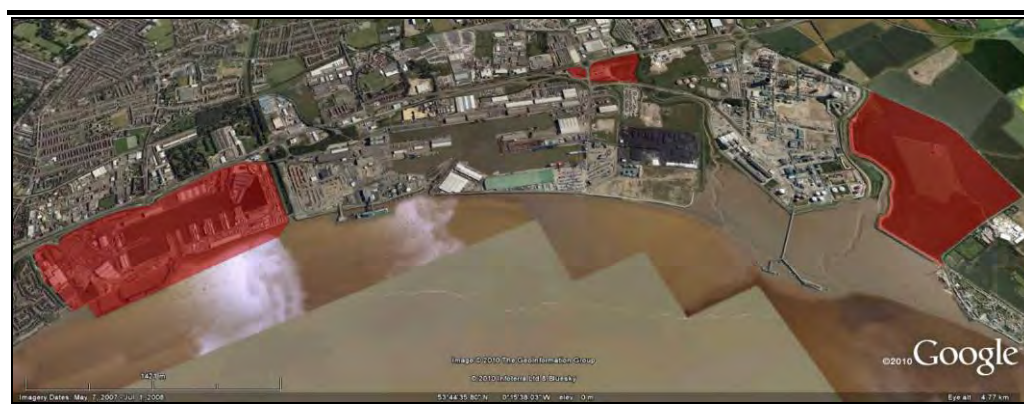
Figure 7.6 Aerial View of Hull
